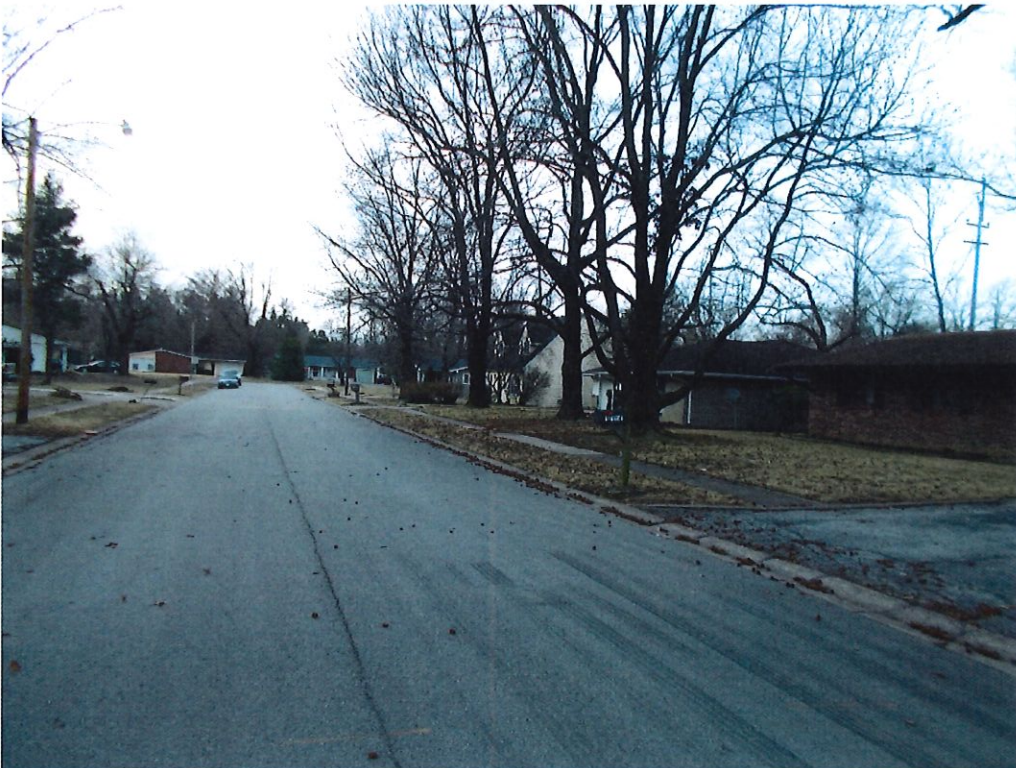
View facing south along South Terrace Drive
