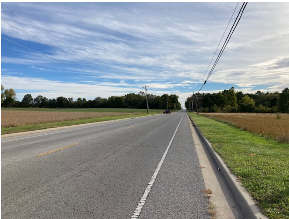
View facing south along New Era Road
