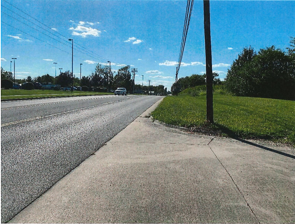
View facing west along East Walnut Street
