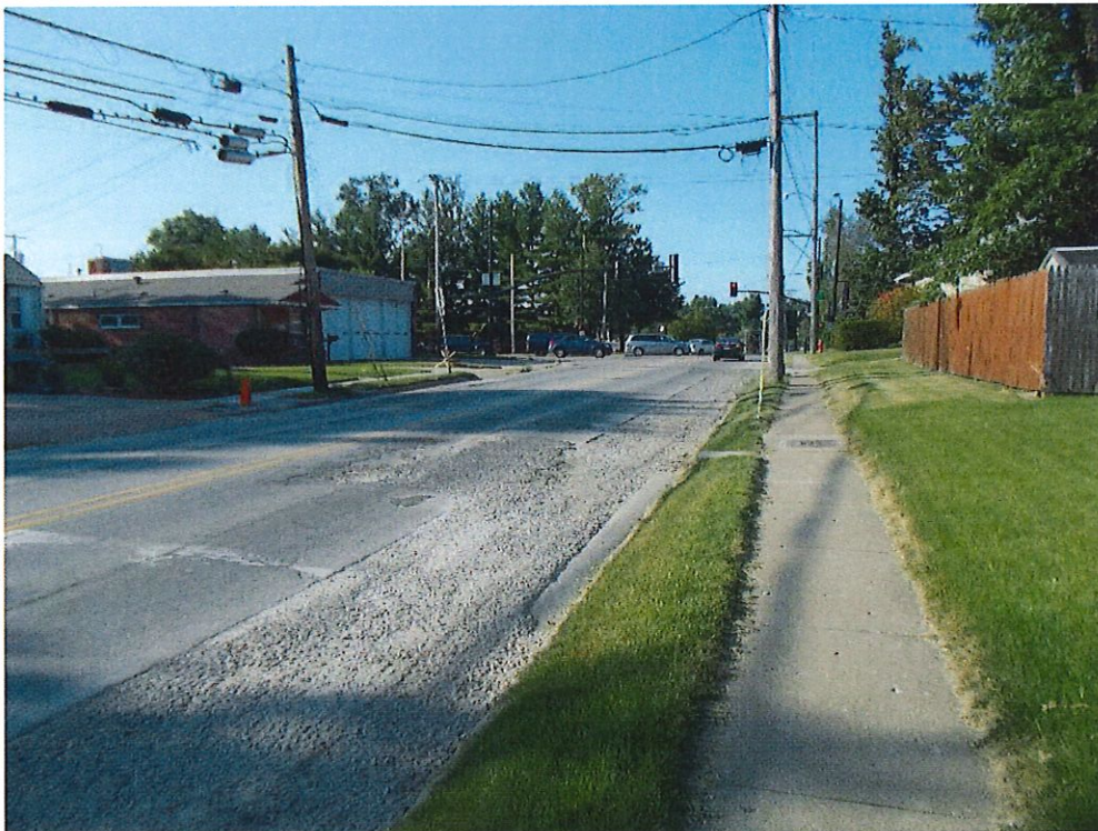
View facing North along South Oakland Avenue
