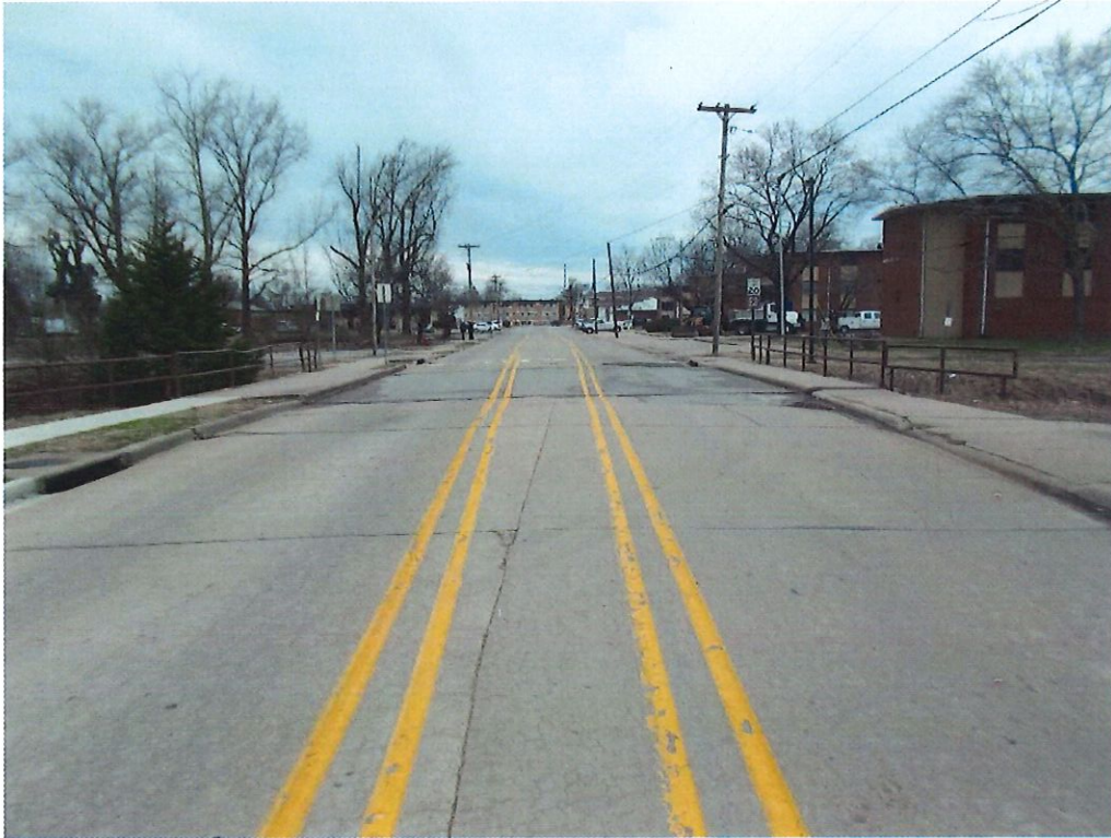
View facing west along East College Street
