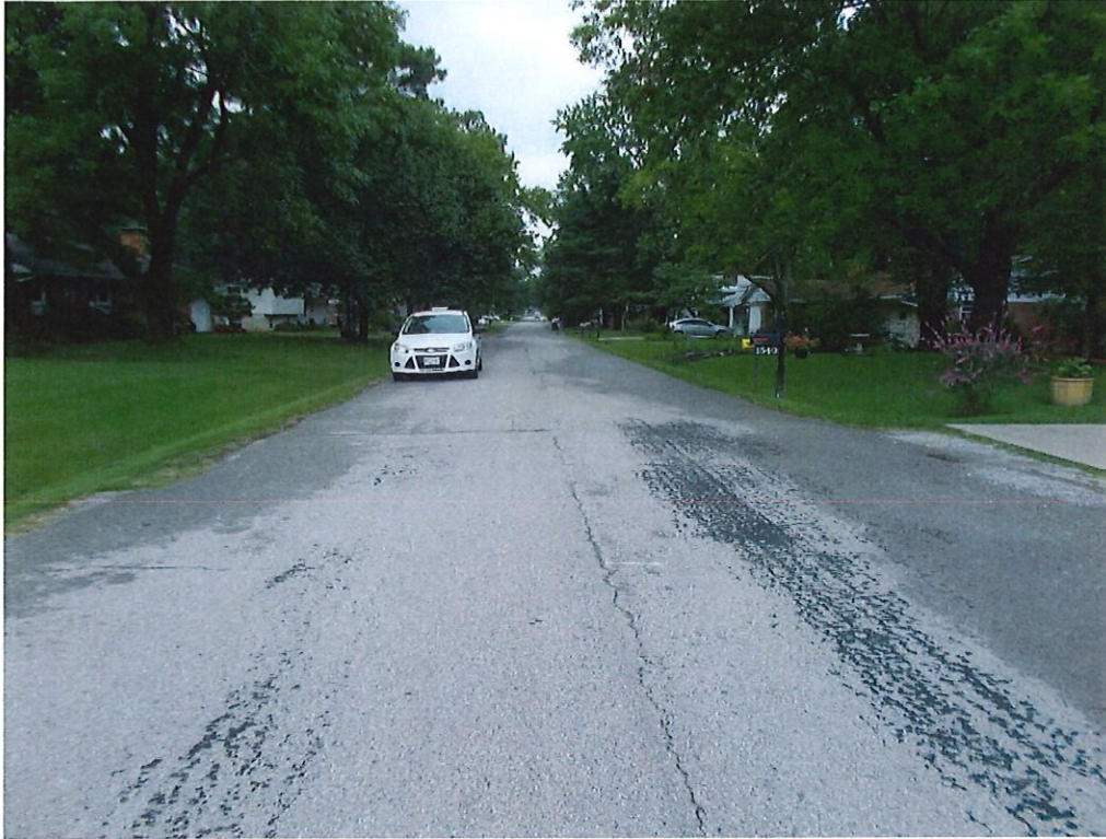
View facing west along East Gary Drive
