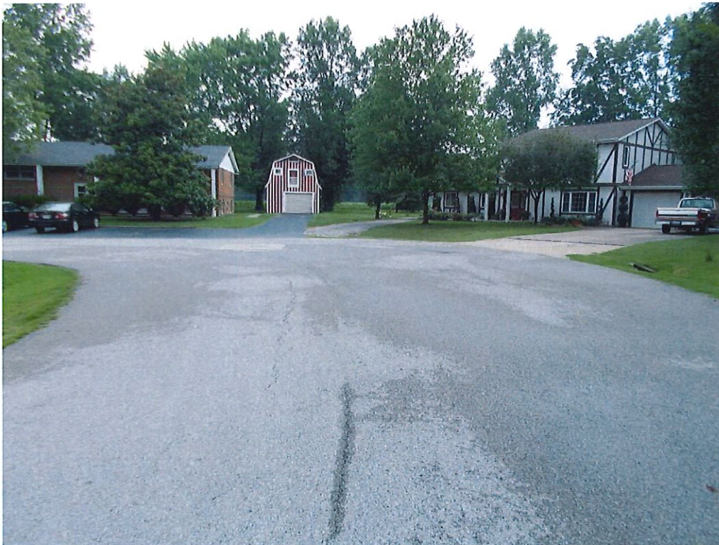
View facing north along South Drury Avenue
