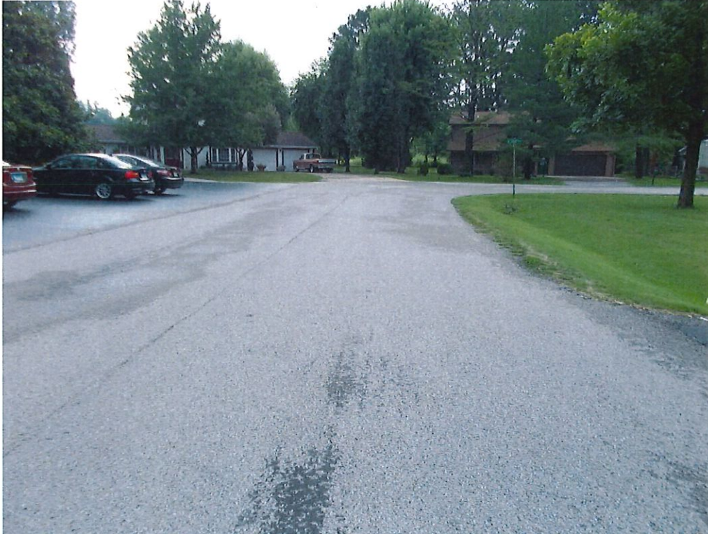
View facing east along East Gary Drive
