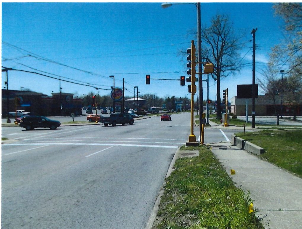
View looking west along West Main Street
