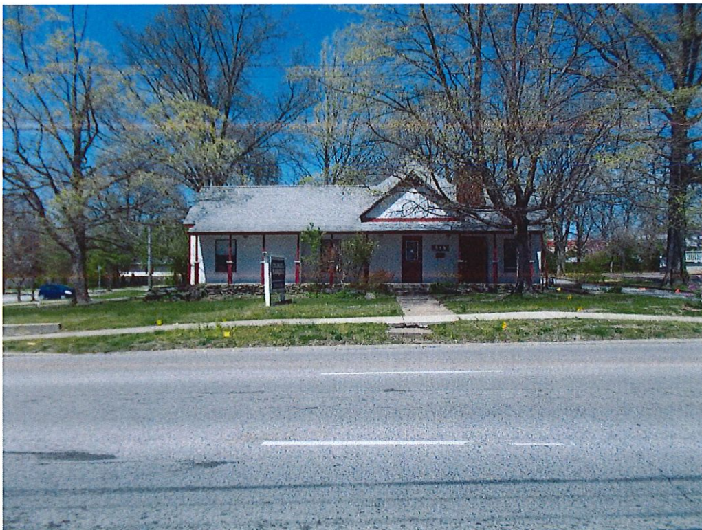
View of 818 West Main Street across West Main Street
