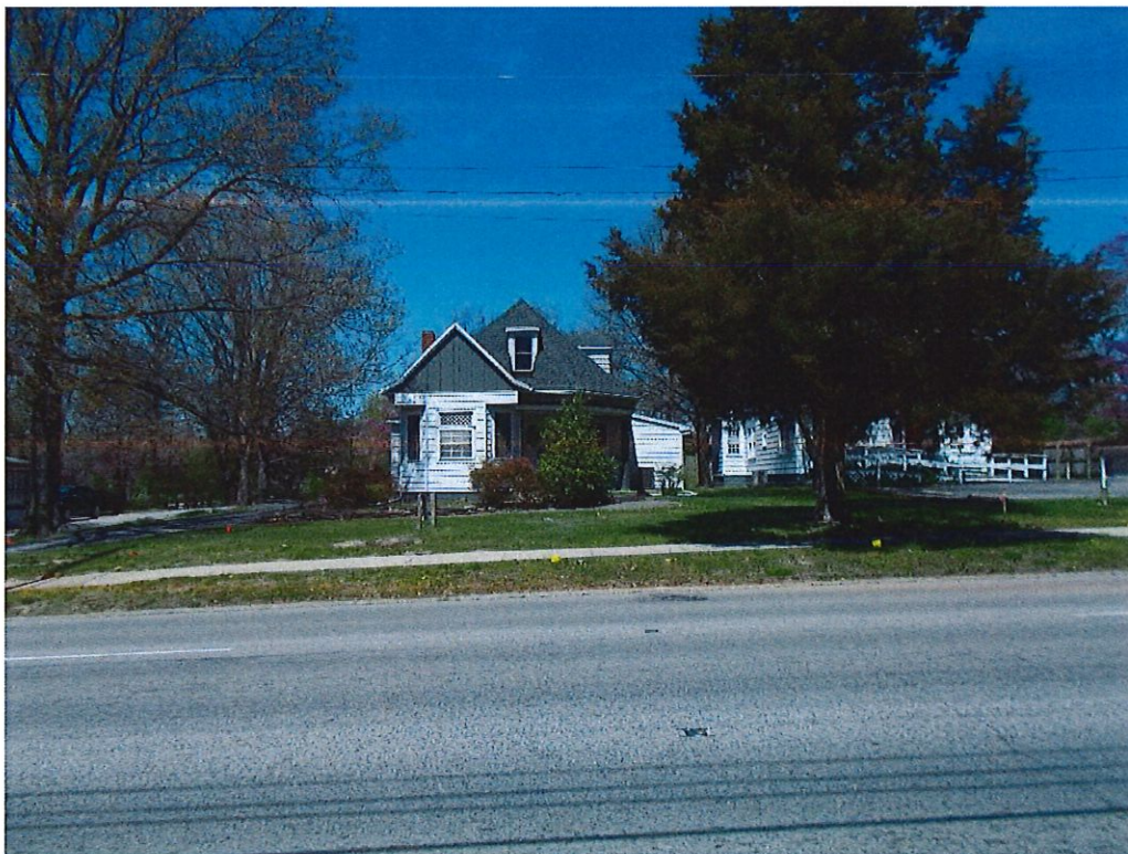
View of 816 West Main Street across West Main Street
