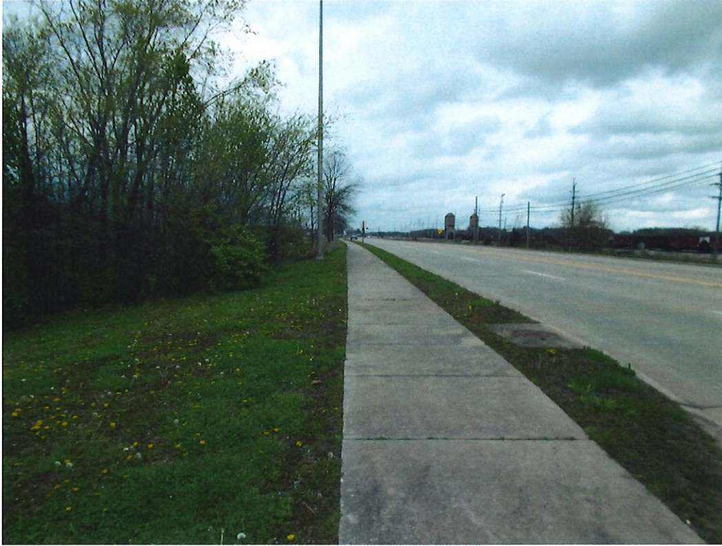
View north along North Illinois Avenue
