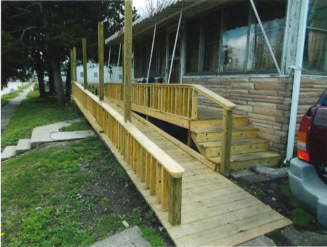
Facing the newly constructed uncovered accessible ramp facing North Washington Street
