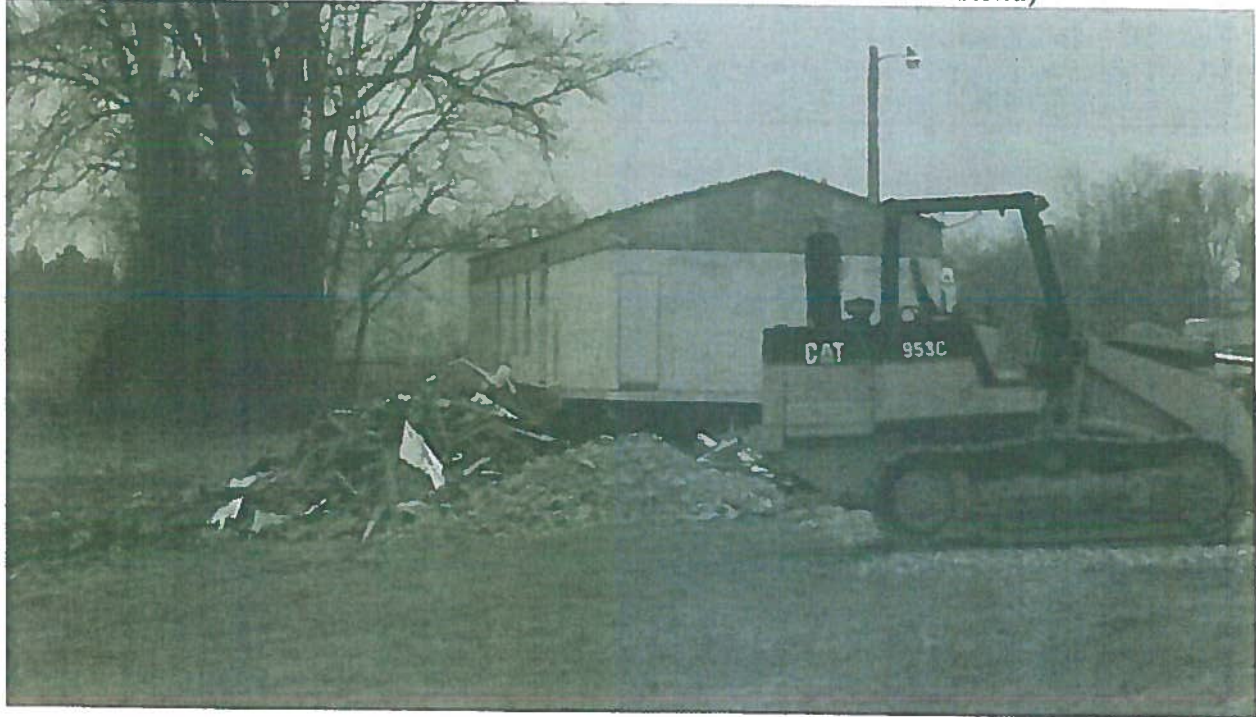
Existing Location, 39 Salt Life Lane (as seen from West Pleasant Hill Road)
